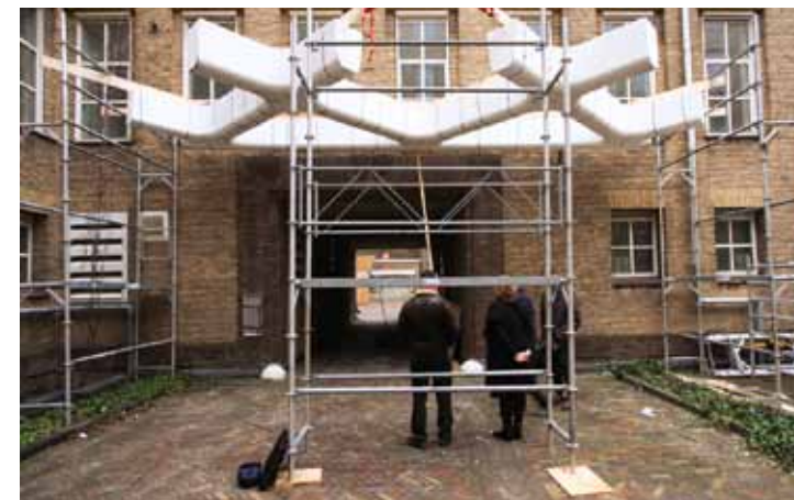
DURING THE DESIGN PHASE, A POLYSTYRENE MOCK-UP WAS HUNG UP AT THE INTENDED HEIGHT TO STUDY THE EFFECT.
