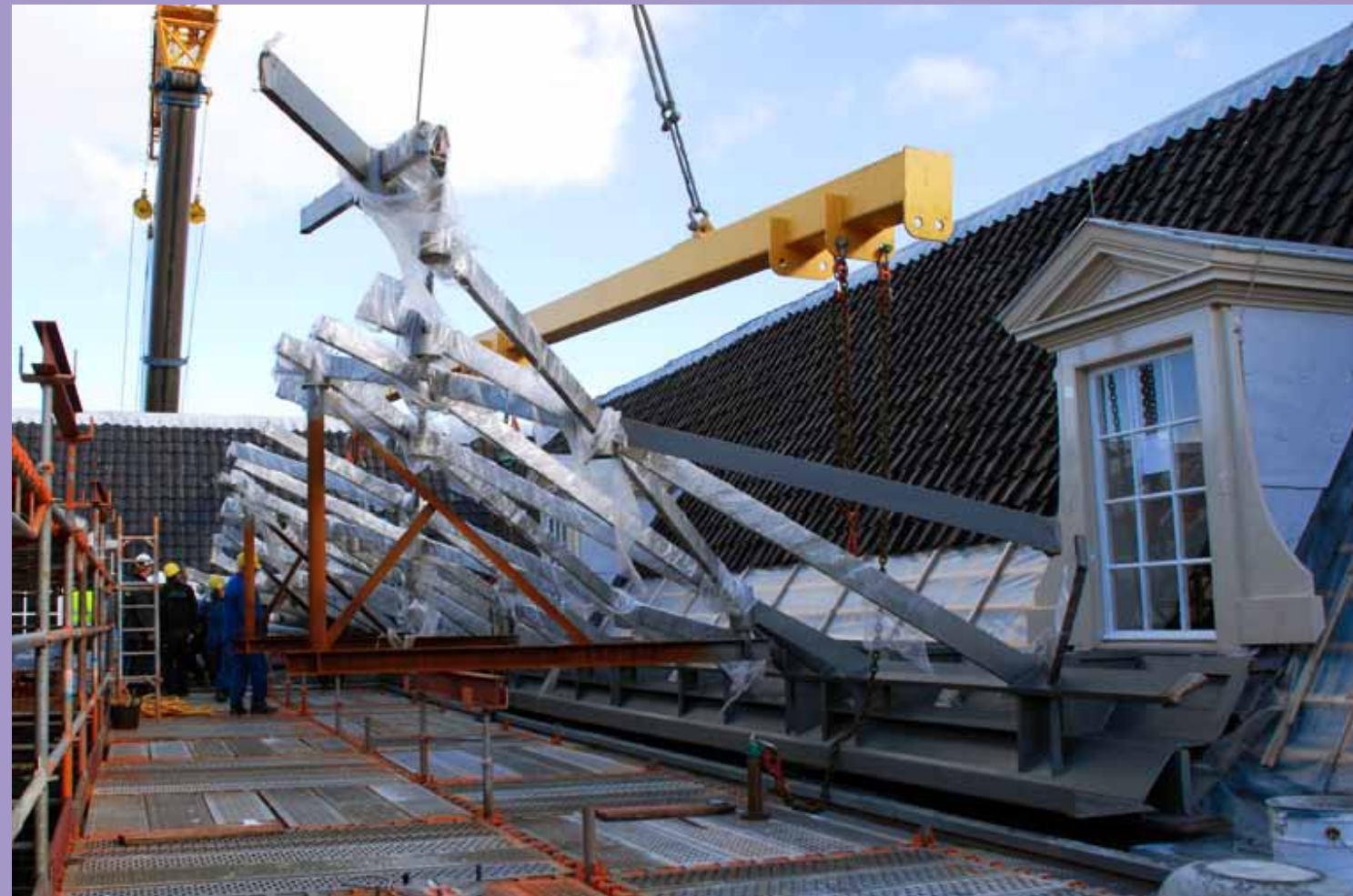
THE ENTIRE STEEL CONSTRUCTION IS IN POSITION AND THE GLAZING BEADS HAVE BEEN FITTED. STEEL GRIDS COVER THE NEW GUTTER.
