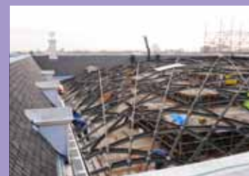
THE ENTIRE STEEL CONSTRUCTION IS IN POSITION AND THE GLAZING BEADS HAVE BEEN FITTED. STEEL GRIDS COVER THE NEW GUTTER.
